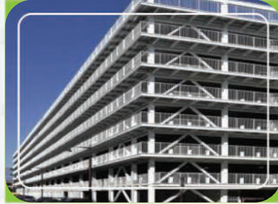
Multistoried Steel Building
